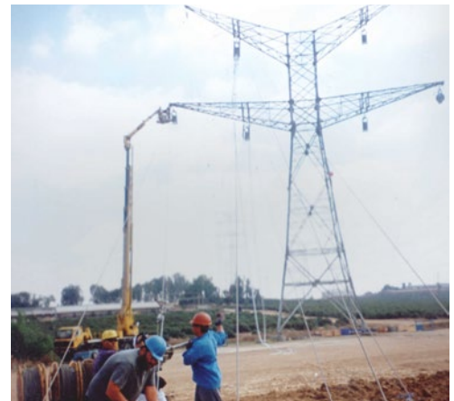
Controlled cable tensioning
